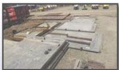
ROAD PLATE & TRENCH BOXES
