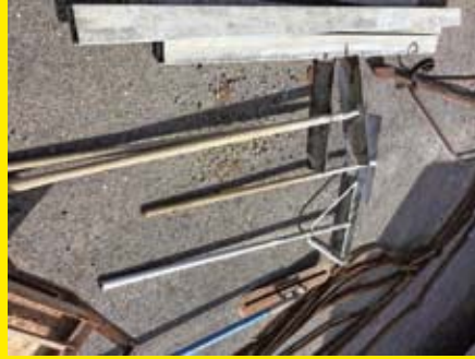
QTY OF CONCRETE & MIX PULLS
